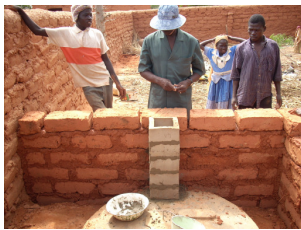
Construction of the ventilation pipe for the slab covering the hole
