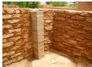
Latrines finished using local materials with defecation hole kept closed at all times with a pipe allowing for ventilation.
