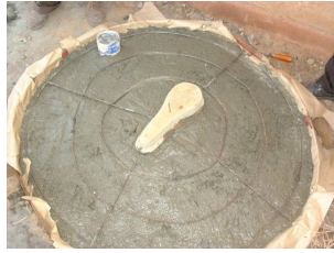
Preparation of the ventilated slab
