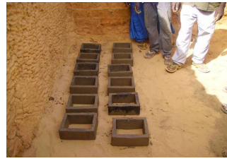
Preparation of the screens for the ventilation pipe
